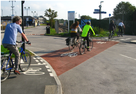
An example of the use of coloured surfacing and cycle symbols to highlight a crossing point.
