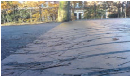
The gentler gradient of a preformed sinusoidal profile ramp.
