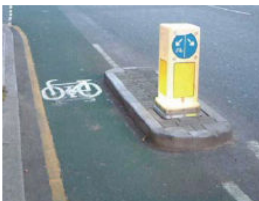
Example of cycle by-pass at a build-out.
