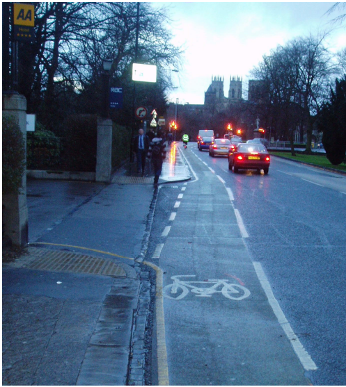
Cycle lane passing side road (diag.1057 is wrongly positioned and should be centrally positioned to the mouth of this minor side road).
