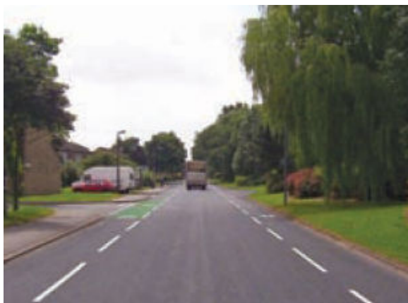
Removal of the centre-line and incorporation of cycle lanes.
